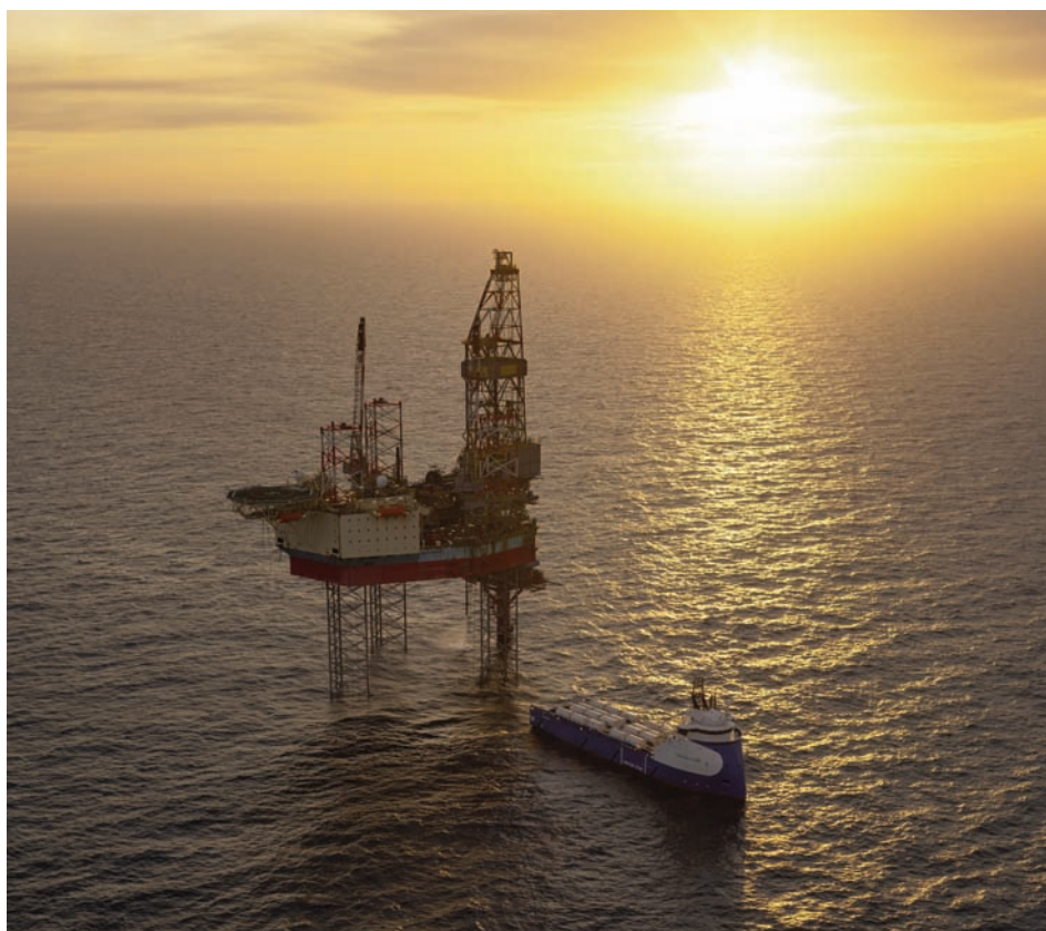
The Greensand Project will have the potential to store up to 8.000.000 tons of CO2 per annum by 2030
