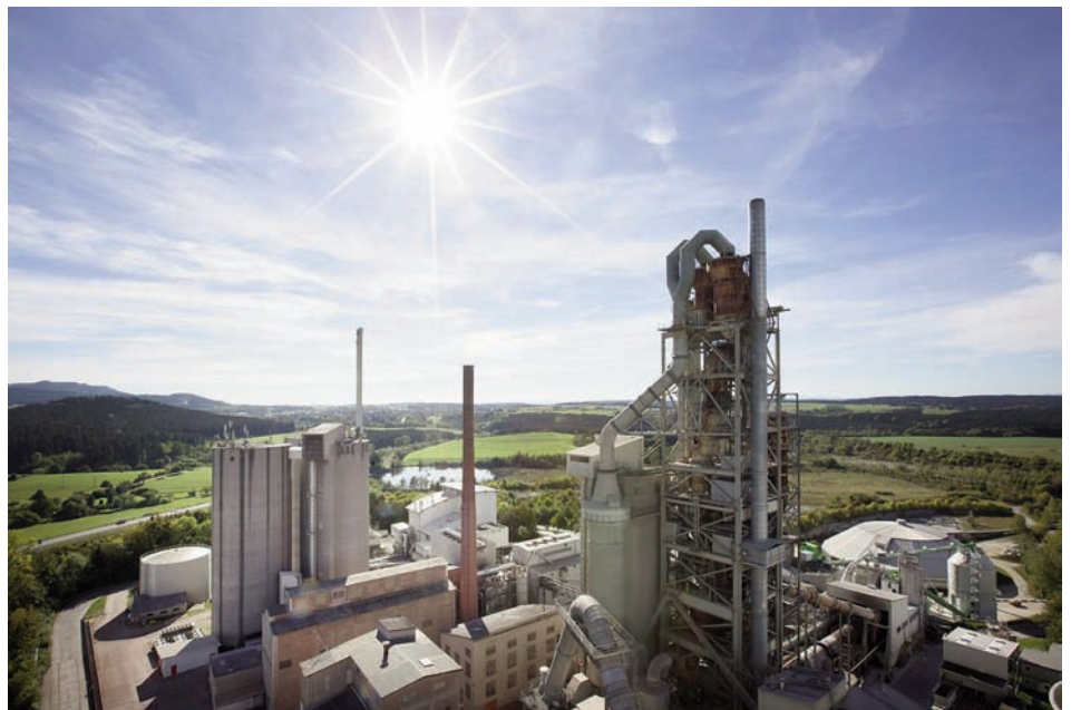
Holcim Group would consider deploying Capsol's carbon capture technology at multiple sites if the Dotternhausen cement plant pilot is successful. Image courtesy of Holcim South Germany
