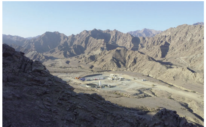
44.01 has started injecting CO 2 at its scaled-up carbon storage site in Fujairah
