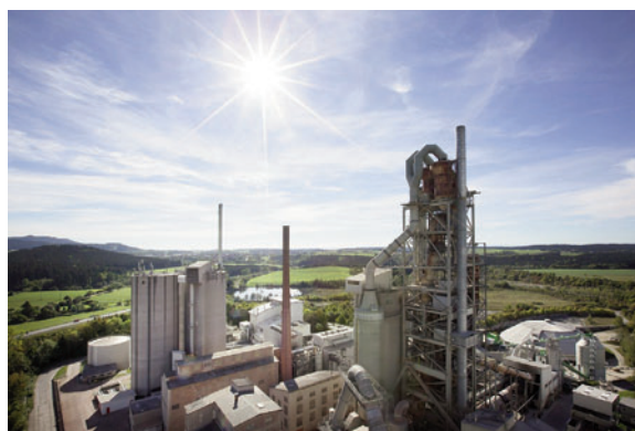
Holcim Group will consider deploying Capsol's carbon capture technology at multiple sites if the Dotternhausen cement plant pilot is successful. Image courtesy of Holcim South Germany
