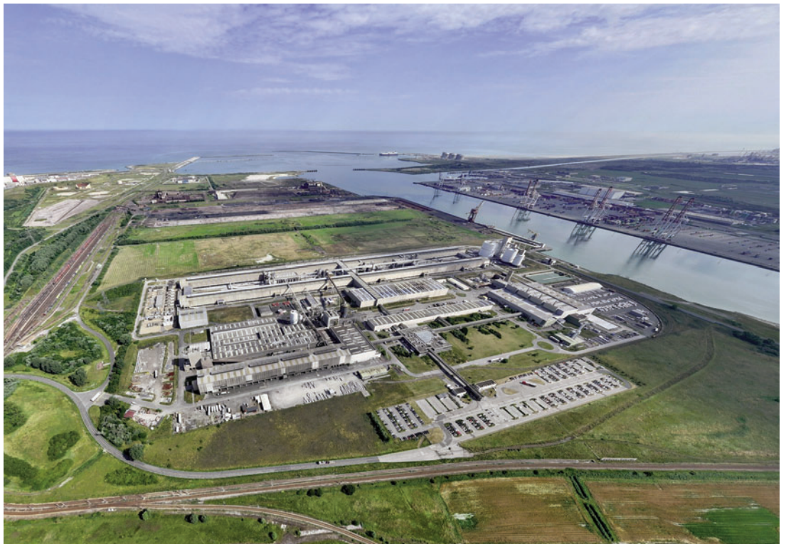
The project will test CO 2 capture on an aluminium plant in real-world conditions. Image: Aluminium Dunkerque
