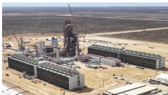
The Stratos project under construction
