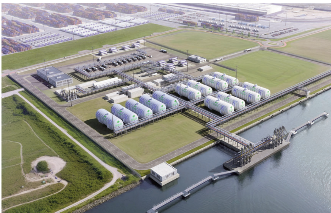
EcoLog Terminal Amsterdam is the world's first commercial-scale liquid hydrogen import and liquid CO2 export facility
