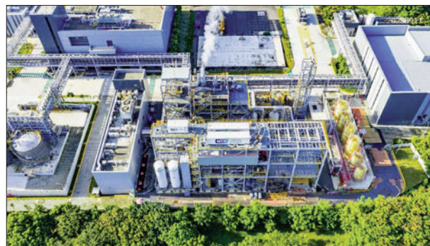
The demonstration facility established by Taiwan Semiconductor Manufacturing Company (TSMC) at the Central Taiwan Science Park is validating the feasibility of membrane-based carbon capture technology in semiconductor manufacturing
