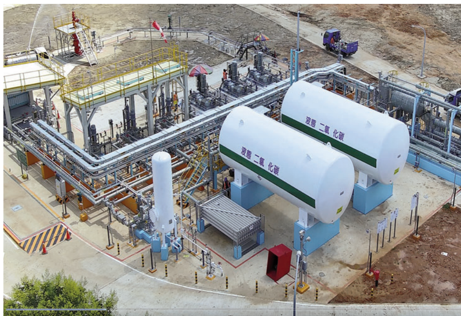
The Tiezhenshan Carbon Storage Pilot Project led by Taiwan's national oil company CPC Corporation completed construction by the end of 2025
