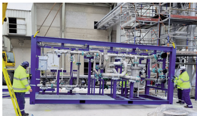
One of the prefabricated modules being installed
